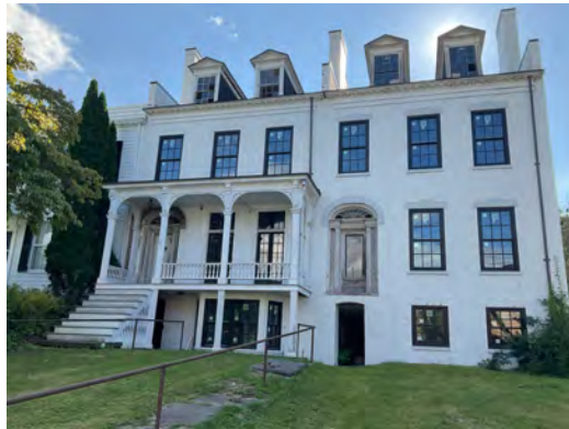
Above: Front of infrastructure improvement
