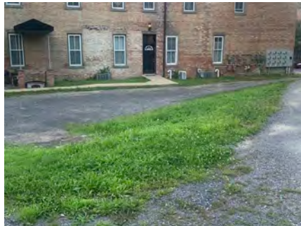
Above: back driveway, needs restoration
