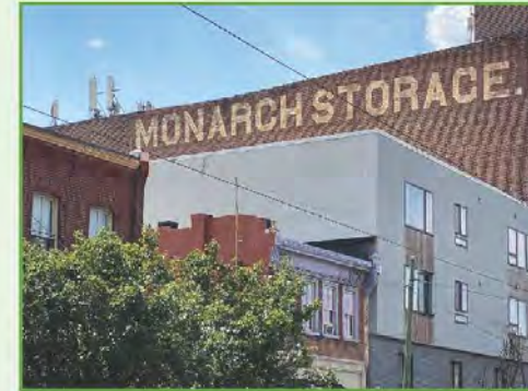
Left: Exposed antennas and stealth antennas cloaked in brick on the roof of a building at 39th Street and Lancaster Avenue, Philadelphia. (Photo: Michael Bixler)
