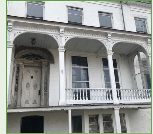
Above: 2-4 Mansion Street's Porch (Photo: Bryan T. McDonald)
