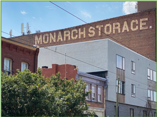
Left: Exposed antennas and steal-thed antennas cloaked in brick on the roof of a building at 39th Street and Lancaster Avenue, Philadelphia. (Photo: Michael Bixler)
