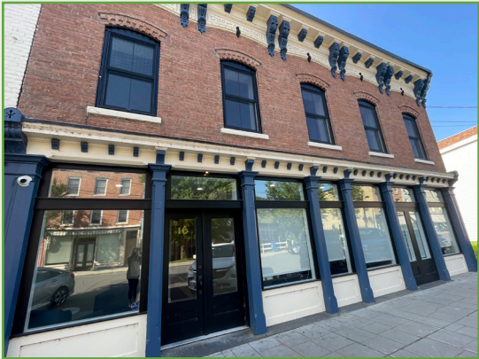
Left: The new windows would follow a very similar pattern to 16 Reed Street. (Photo: National Bank of Coxsackie)
