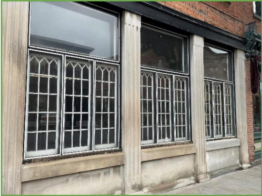
Left: Current Reed Street facing windows (Photo: National Bank of Coxsackie)
